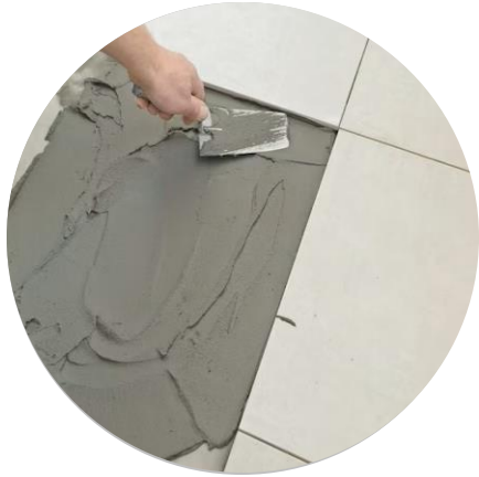
Tile fixing with cement
