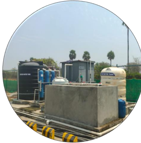
STP Installation & Treated Water Reuse
