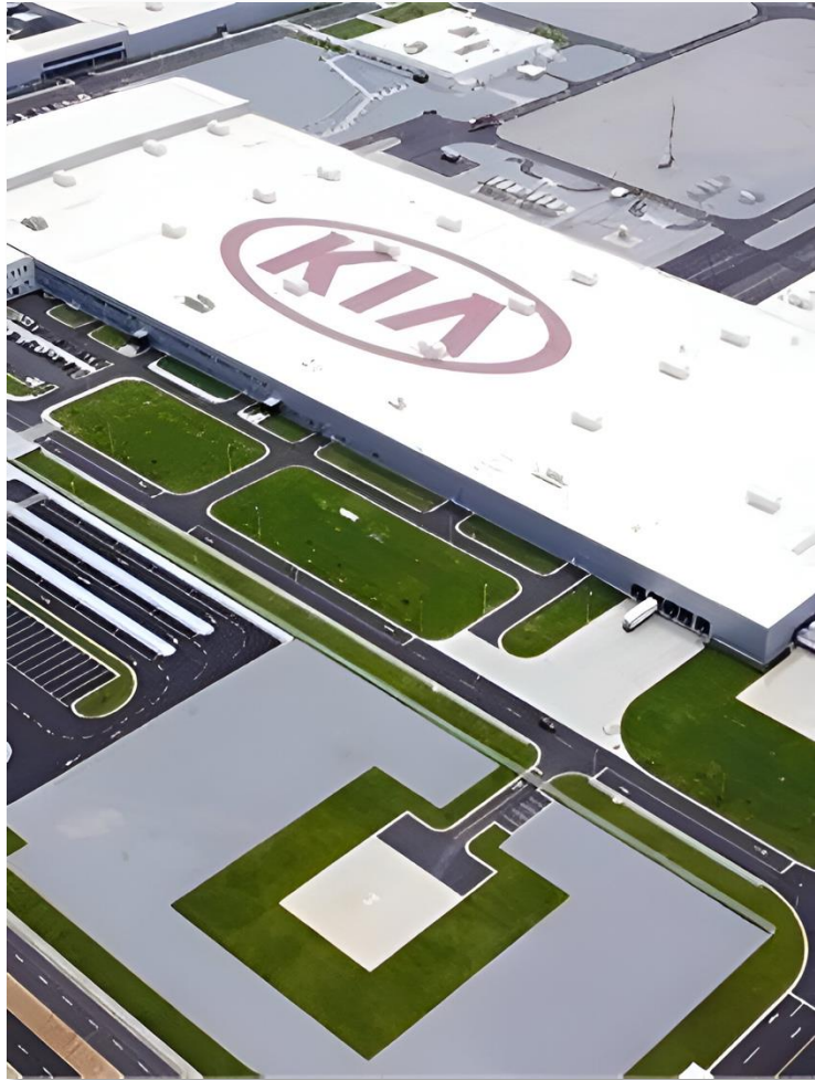
KIA Motors Mfg. Facility (One of Largest Industrial Roof with preformed TPO Membrane w/p project)
