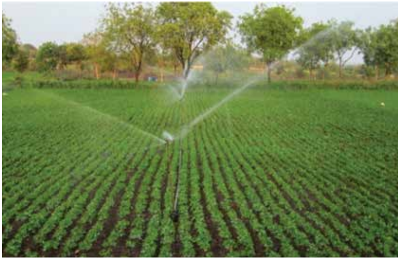
(Drip irrigation installation at farmer field)
